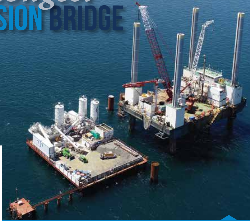
COMPLETE VIEW OF THE CHACAO CHANNEL, JACK UP BARGE AND SERVICE PLATFORM
