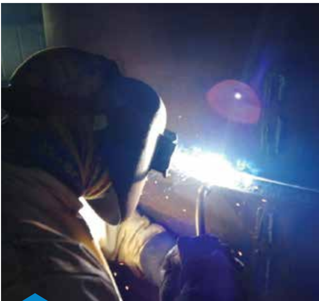
WELDING PROCESS OF THE PERMANENT STEEL CASING
