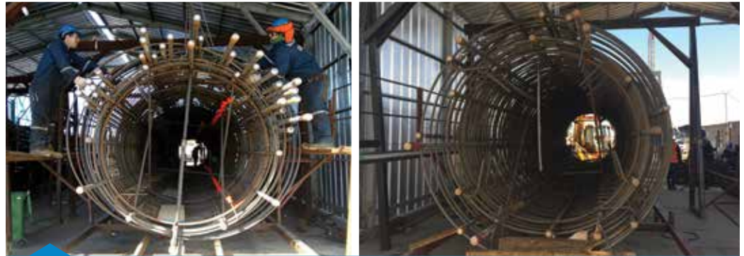
REBAR CAGES AREA
