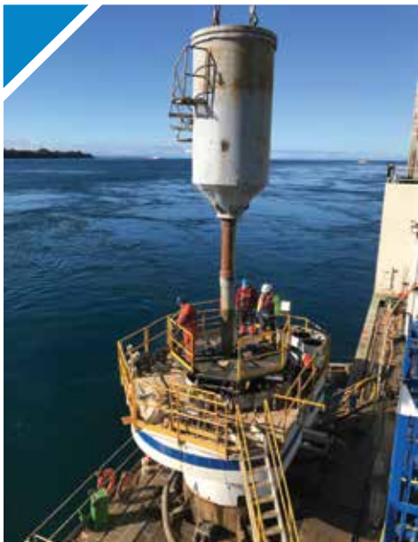
CATAPULT FOR THE STEEL CASING LIFTING
